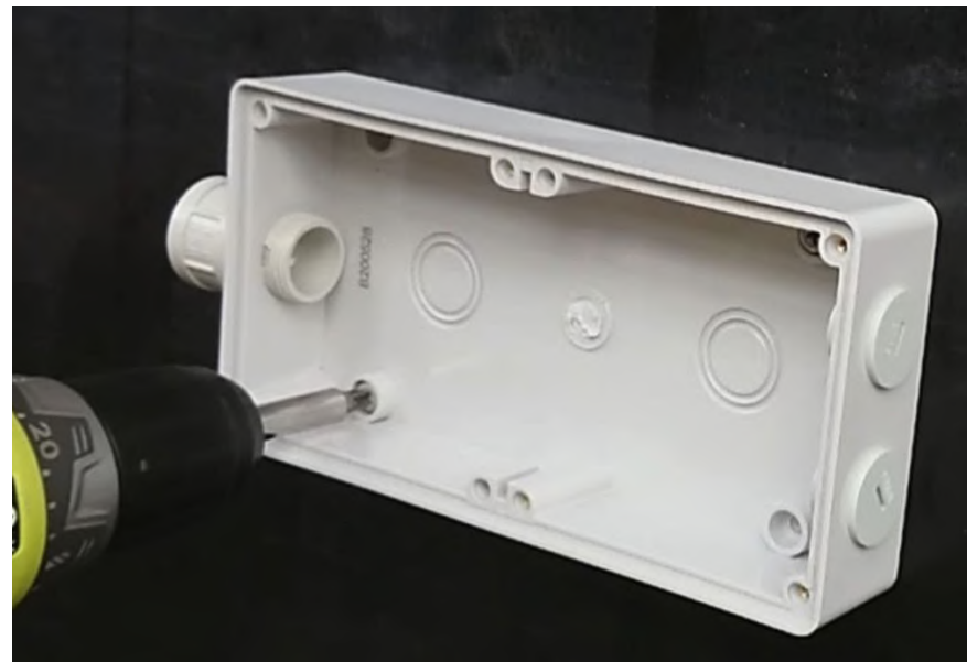
1 - Mount Enclosure Base to Wall
